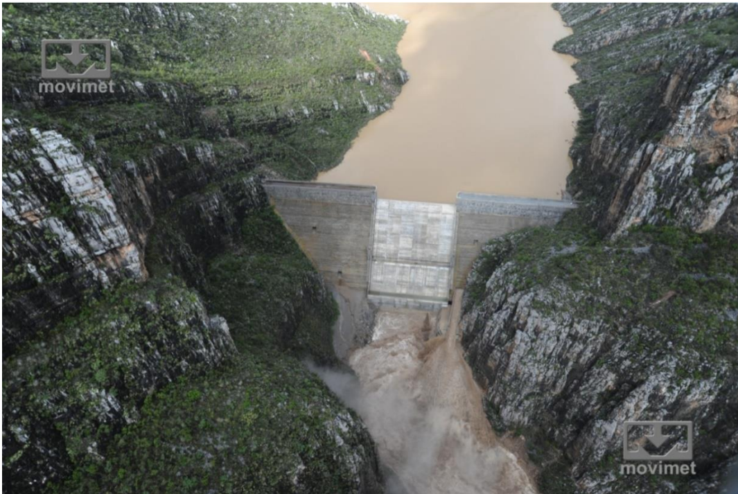
Figure 16. Rompepicos Dam at the “Corral de Palmas” site operating during Hurricane Alex storm event in 2010. (Source: Movimet)
